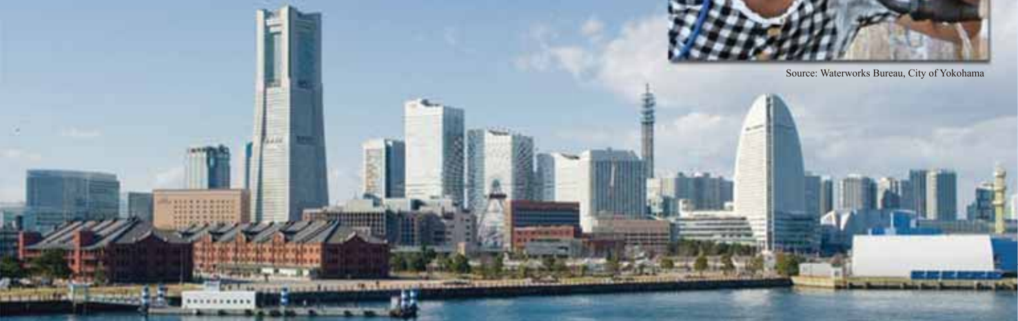
Source: Urban Development Bureau, City of Yokohama
