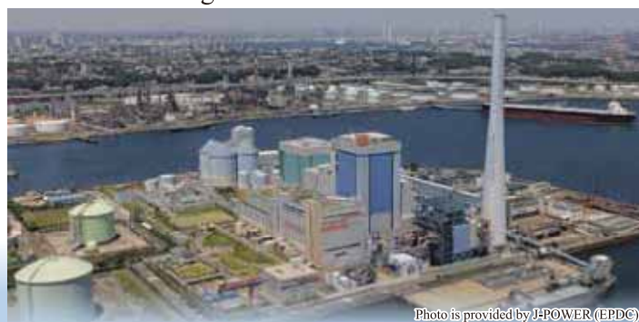
Isogo Thermal Power Plant
